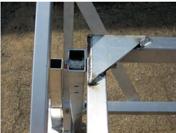
This step may require the help of a partner, but can be done by a single individual if need be. Using the 1/2" x 4" bolts attach the bed frame to the top of the h-brace hinges. Tighten down the bolts by using the 1/2" jam lock nuts. Repeat this step for all four corners.
