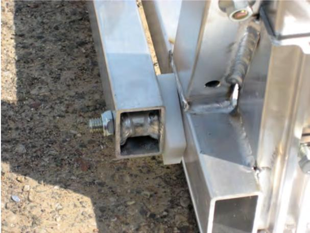
Using the 1/2" x 4-1/2" bolts attach the h-brace to the bottom of the lift side using the 1/2" jam lock nuts. Be sure that the nylon spacer is placed between the hinge and side frame like the picture in the left. Repeat this step for the remaining h-braces.
